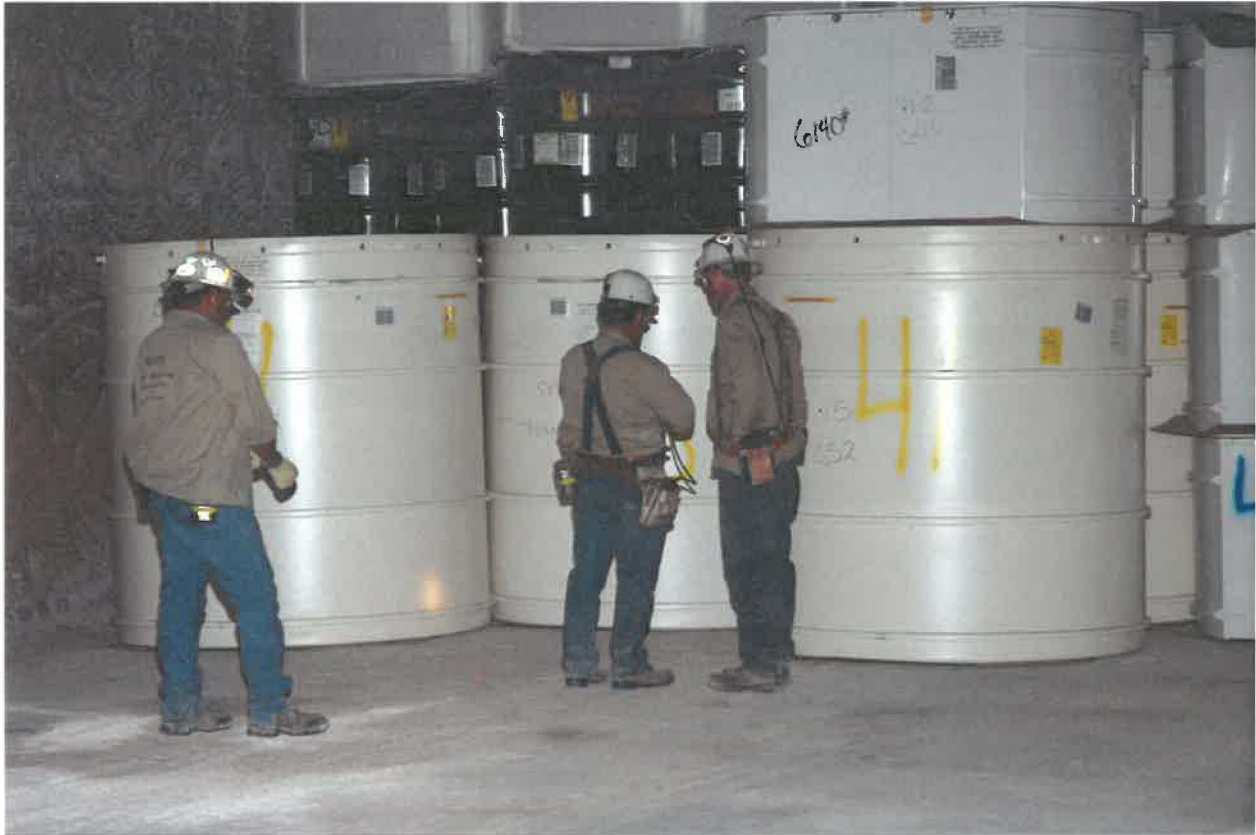
Figure 1. CH Waste Packaging Configurations in the WIPP. The black drums in the picture are 55-gallon drums shrink wrapped together into a 7-pack, and the containers on the floor are TDOPs. A SWB is placed on top of a TDOP on the right side of the picture. At the top of each stack is a supersack of MgO.
